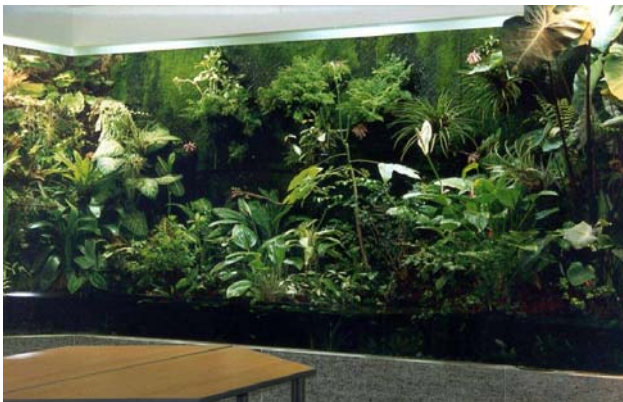
Figure 3.0: Small Scale Biofilter (10m 2 biofilter at Canada Life Centre, CLER)
